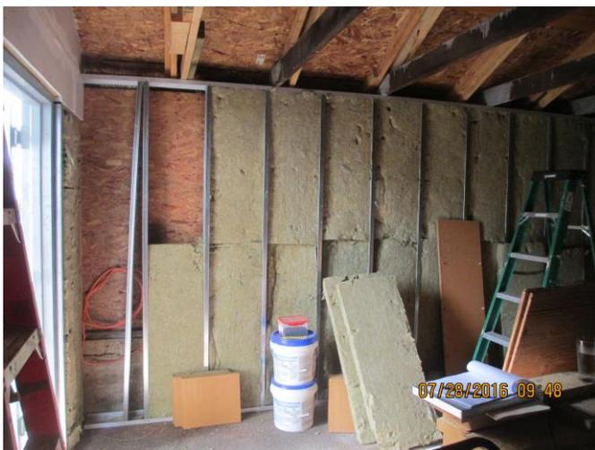
Typical Soundproofing of Interior Wall
